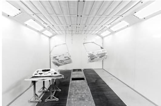
Easily installed into any high bay light fixture, newer models rely on LED technology and therefore do not require special electronics or rewiring. The LED T-8 design also offers more sustainable operation than a standard fluorescent lighting package, reportedly saving up to 40% on electricity costs.
